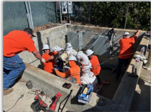
Pump replacement and drywell rehabilitation.
