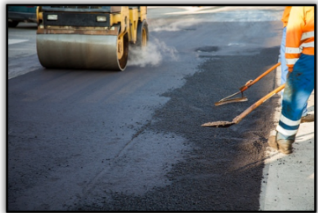
Asphalt being applied after gravity pipeline replacement.
