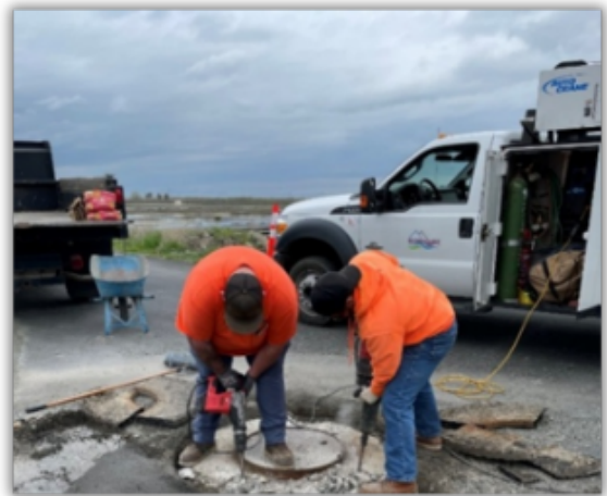
Manhole frame and cover replacement.
