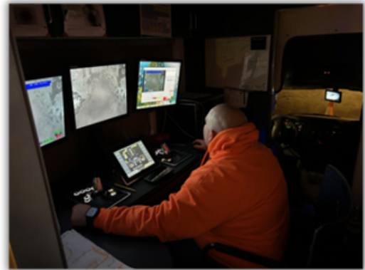
Closed Circuit Television operating station.
