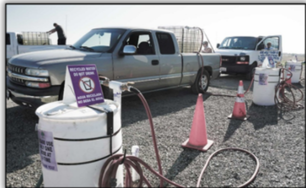
Recycled Water Fill Station.
