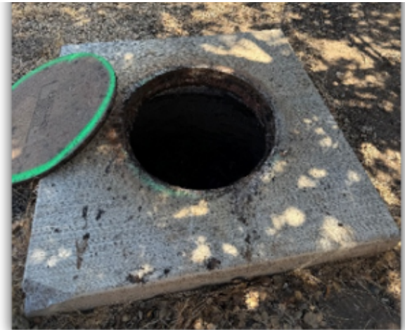
Manhole cover and frame.
