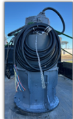
Sludge Pump after rehab.
