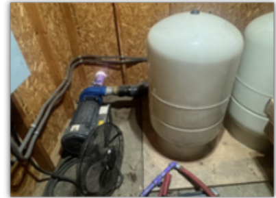
Installation of a recycled water pump station.
