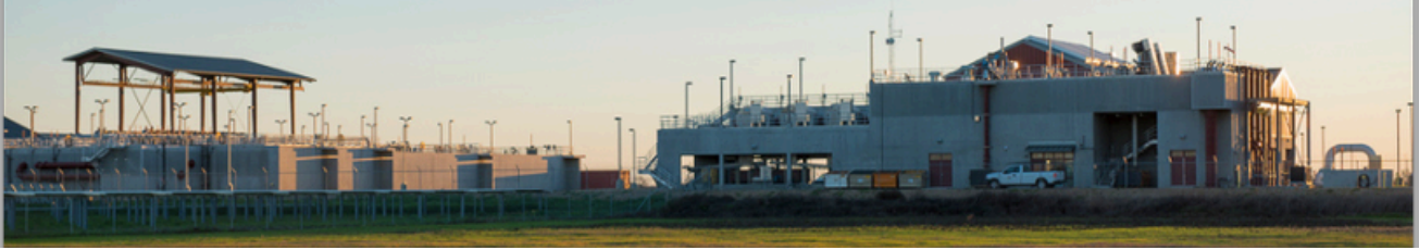
Water Recycling Facility at Ironhouse Sanitary District.
