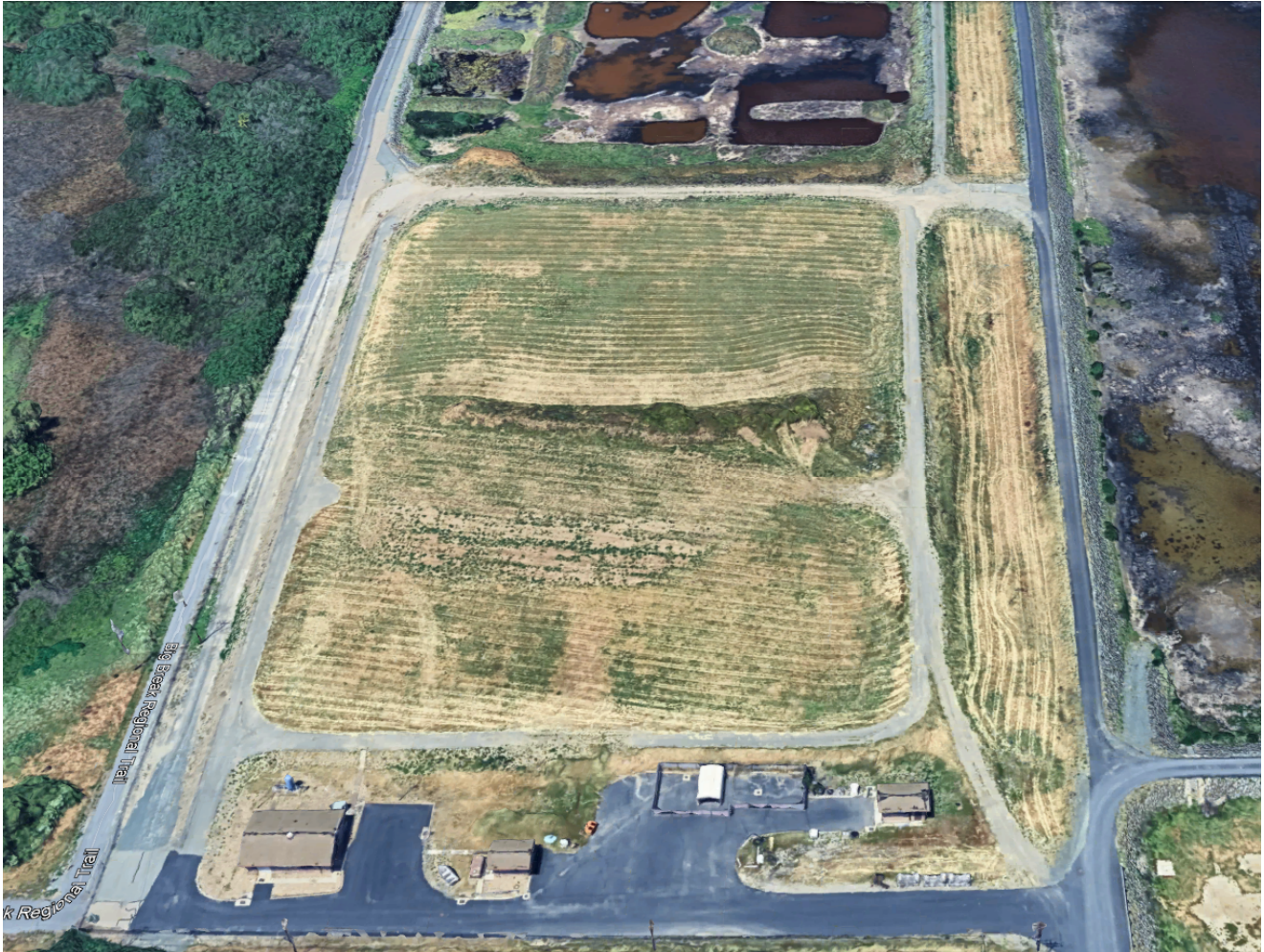
Figure 18.2. Original WWTP Site
