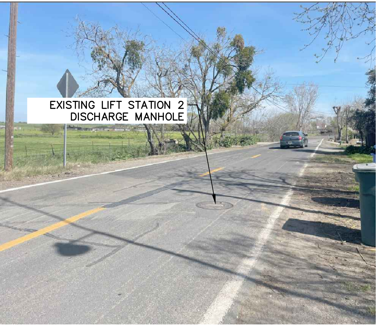
PHOTO 1 - MANHOLE PROXIMITY 1 NOT TO SCALE
